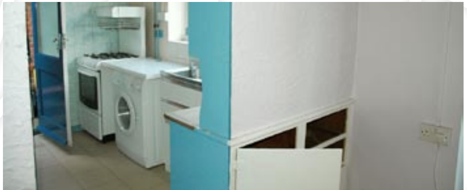
Kitchen Refurbishment – Before
