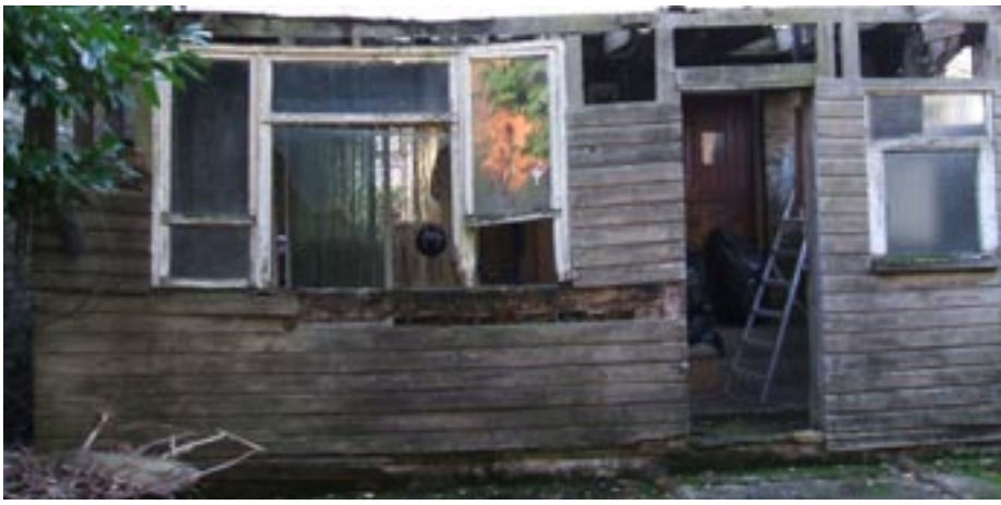
Major Refurbishment – Before
