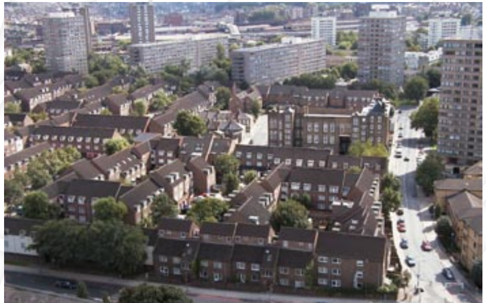
Kambala Estate, London - Window Replacements and External Redecoration
