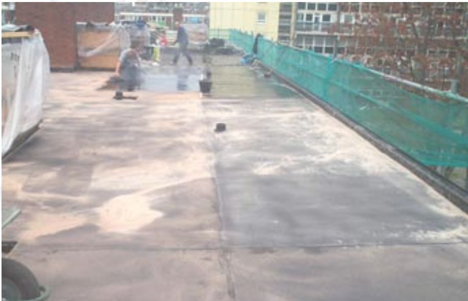
Jagger House, London - Asphalt Re-Roofing
