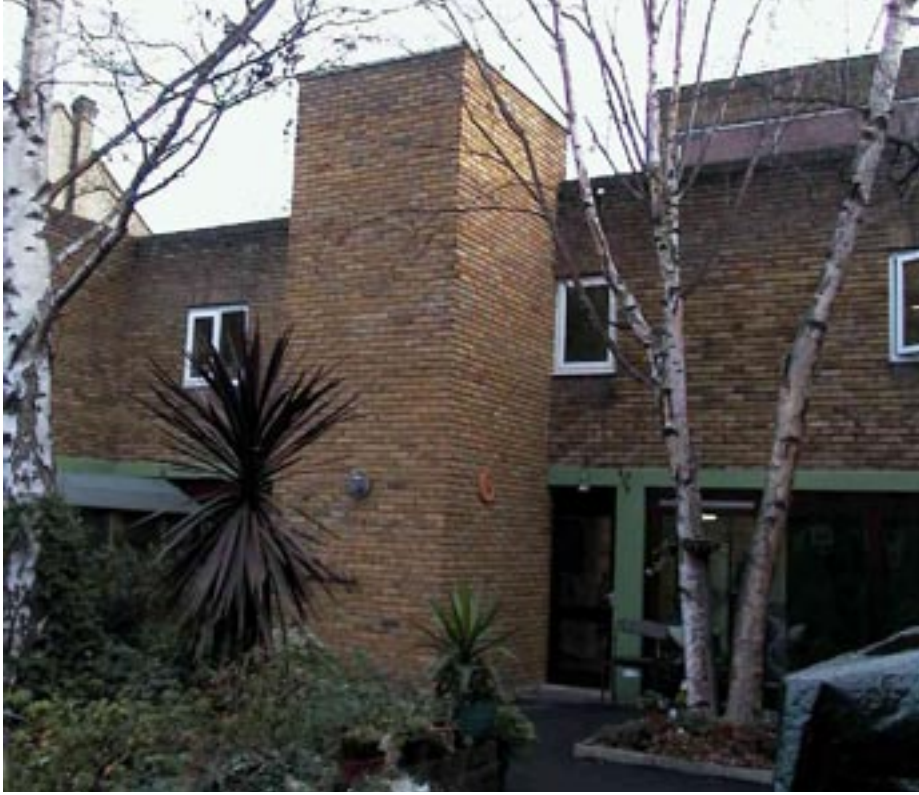
Hill Lodge, London - Construction of New Lift Shaft
