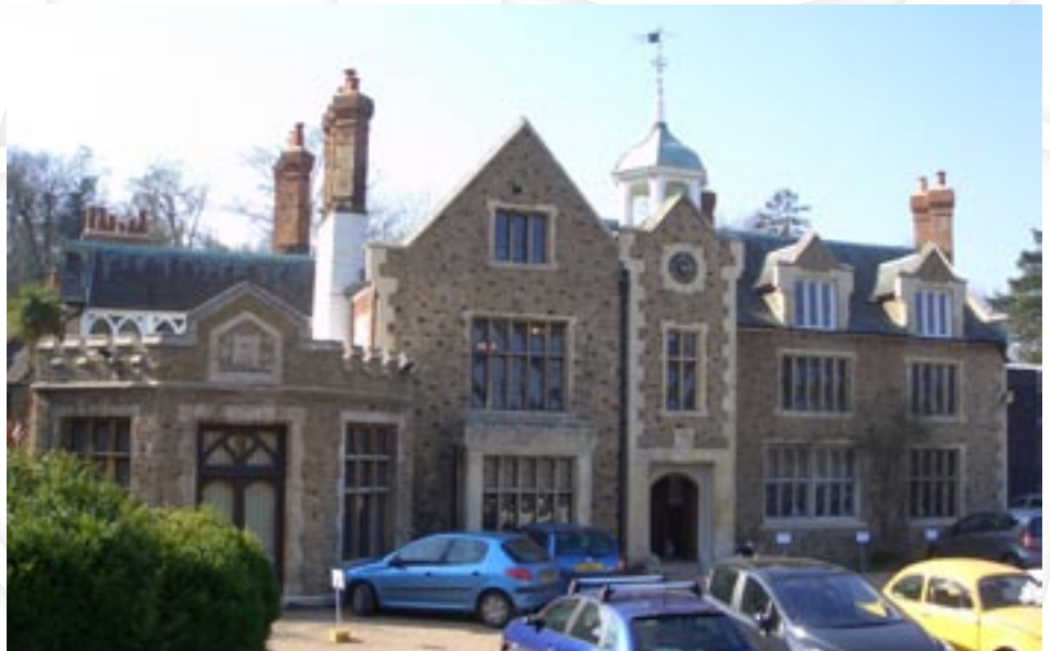
Guildford College of Law - Condition Survey & Planned Maintenance Report
