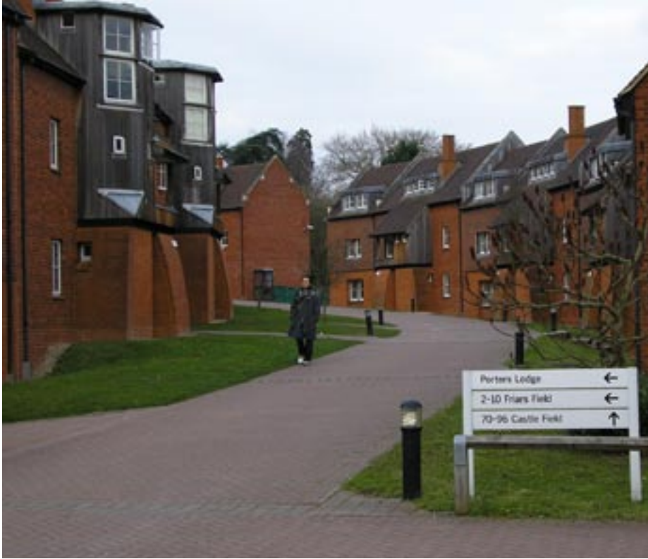
University for the Creative Arts - Defects Survey on External Wall Cladding
