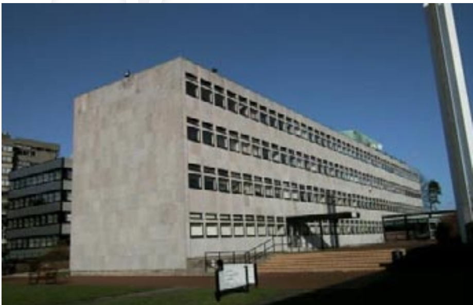
University of Southampton - Defects Survey on Stone External Wall Cladding
