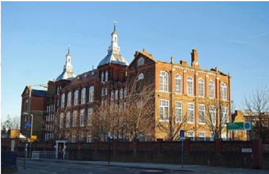
Smallwood School, London - External Redecoration and Repair Works
