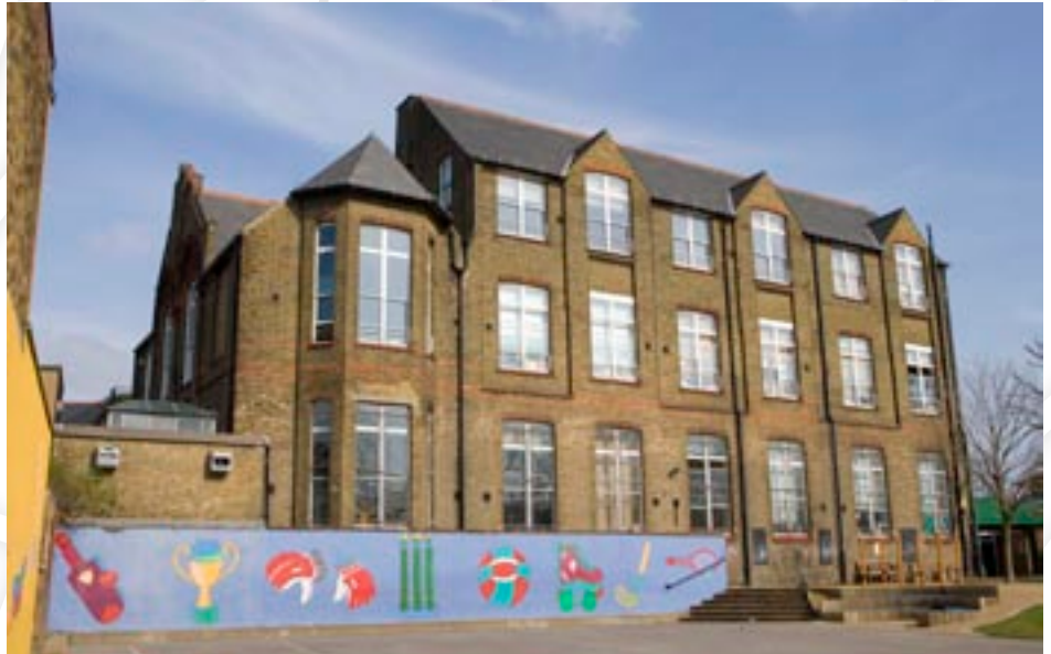
Wilberforce School, Westminster - Window Replacement and Re-pointing Works
