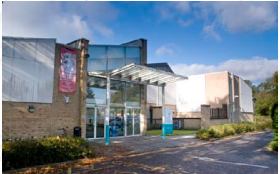
Herons Leisure Centre – Defects Reports and Remedial Works
