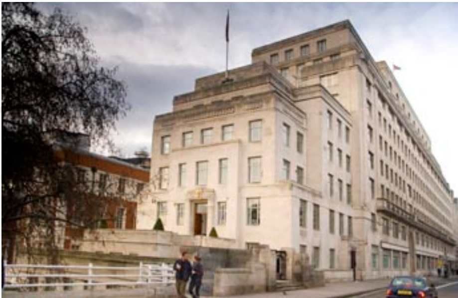
Duchy of Lancaster House – Roof Repairs
