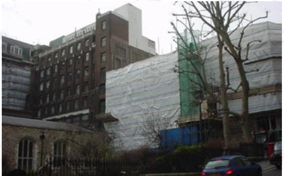
The Strand – Refurbishment and Party Wall Works
